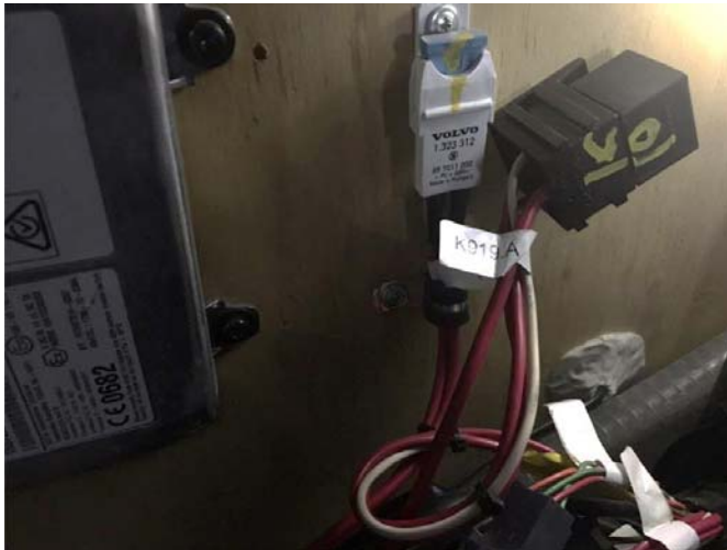
FIGURE 2: RELAY K919 LOCATED UNDER THE DRIVER AREA FLOOR
