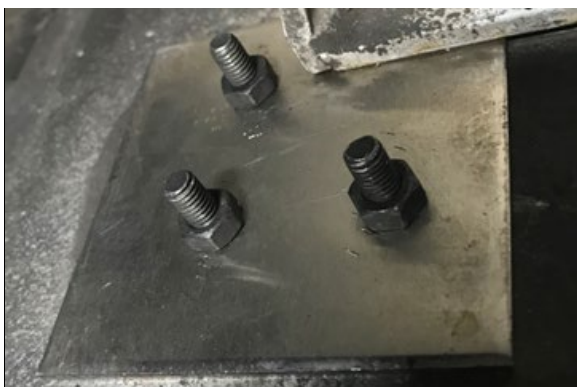
FIGURE 22: REINFORCEMENT PLATE INSTALLED
