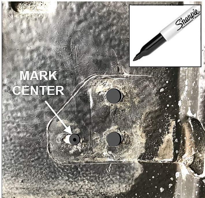
FIGURE 16 : MARKING THE PLATE WITH A SHARPIE PEN
