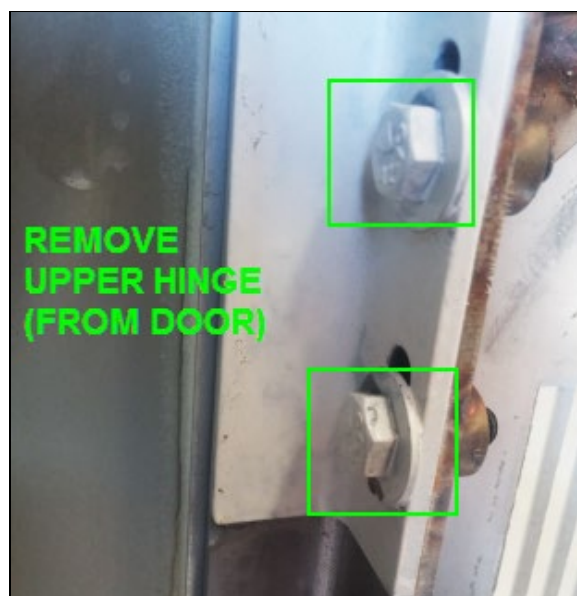
FIGURE 4 UPPER HINGE REMOVAL DOOR SIDE
