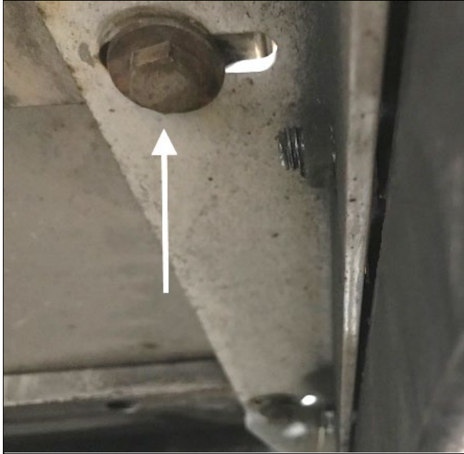
FIGURE 14: BATTERY TRAY BOLT (3X UNDERSIDE)
