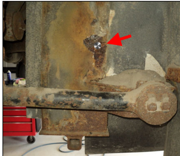
FIGURE 6: CLEANED SPOT ON STRUCTURAL MEMBER
