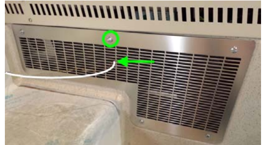
Insert the 2 nd sensor in the defrost return air intake, under the screw found at the center.
