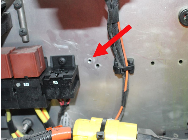
FIGURE 27: INSTALLATION DE LA BASE DE RELAI
