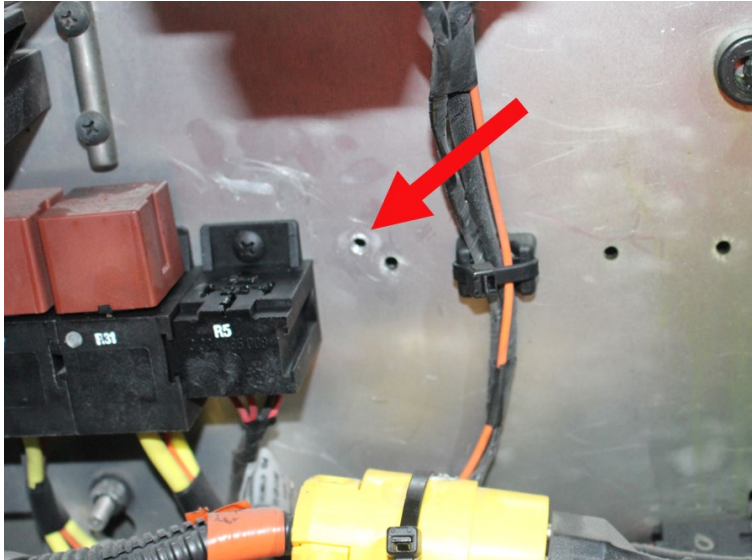
FIGURE 38: INSTALLATION DE LA BASE DE RELAI
