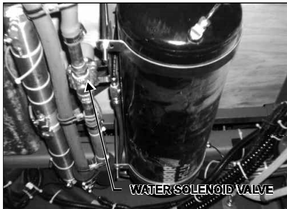
22049 FIGURE 30: CEILING OF THE SPARE WHEEL COMPARTMENT
