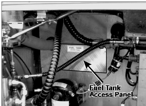
FIGURE 4: FUEL TANK ACCESS PANEL LOCATION
