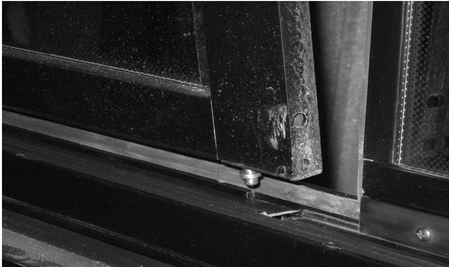
FIGURE 42: DISENGAGING THE BOTTOM OF THE SASH
