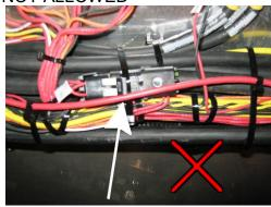
Possible contact or rubbing against screws, edges, etc.
