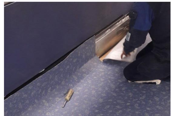
20. Press the linoleum to ensure the adhesion.
