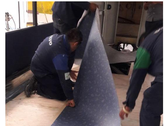
19. Make cuts as required in corners and joints to ensure sealing under the rail and without of bends.
