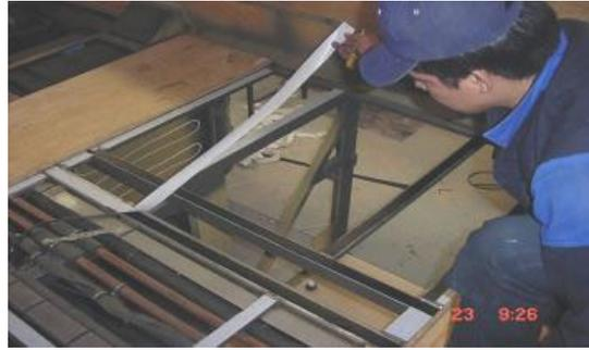
6. Apply Sika Flex on the frame on both sides and in the luggage compartment area.
