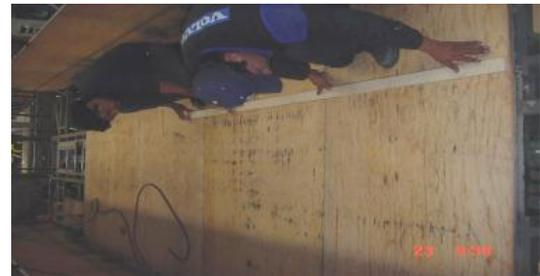
9. Drill holes on the marked places and install the cross recessed sunk screw.
