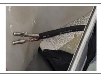
12. Install the harness on the sensor.
