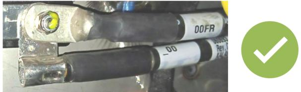
Figure 5: CORRECT INSTALLATION
