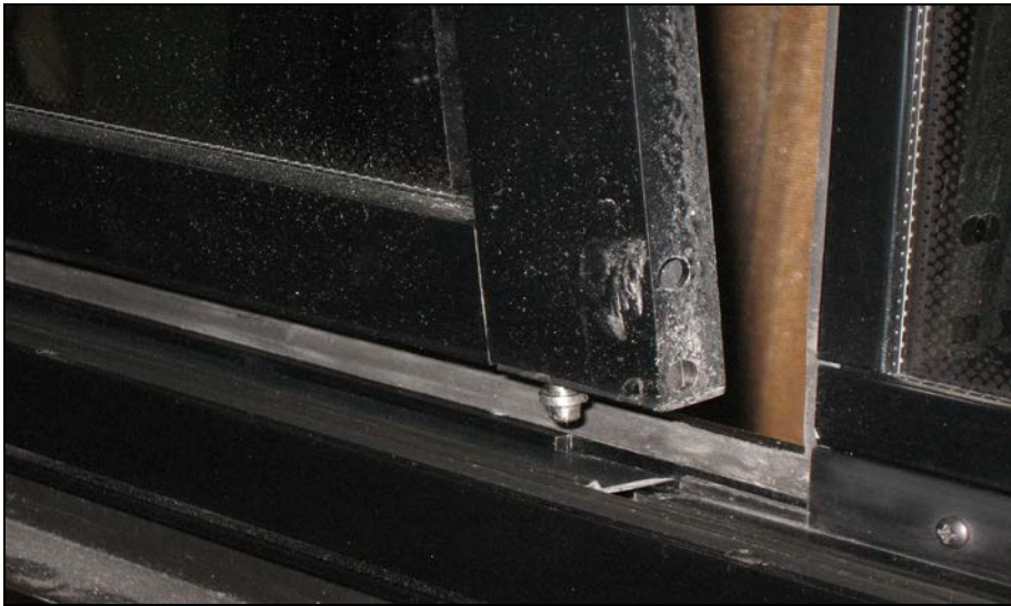
FIGURE 65: DISENGAGING THE BOTTOM OF THE SASH
