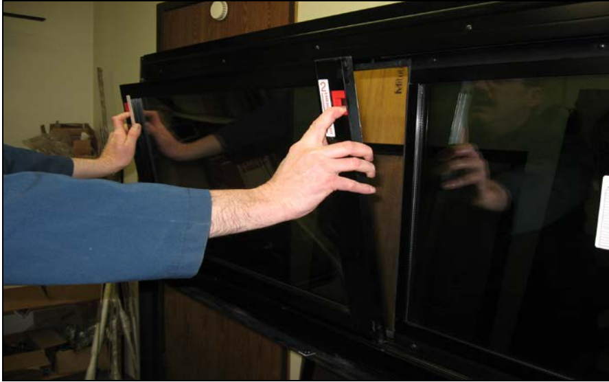
FIGURE 64: REMOVING THE SASH
