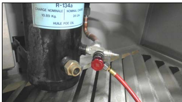
FIGURE 78: RECOVERY UNIT CONNECTED TO RECEIVER SERVICE PORT
