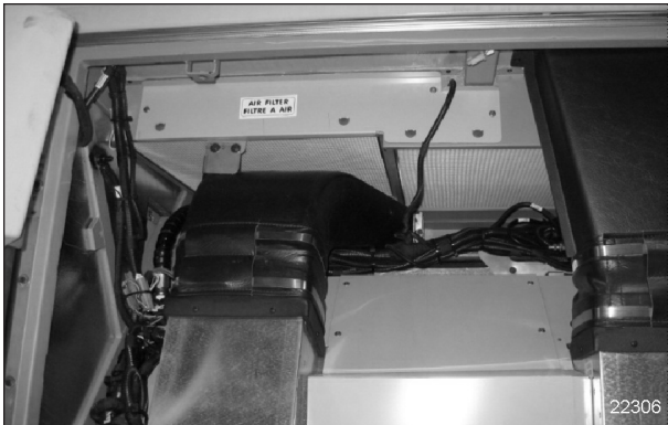
CABIN AREA AIR FILTER REMOVAL
