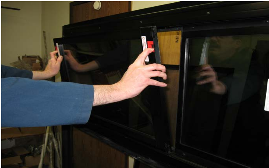
FIGURE 50: REMOVING THE SASH
