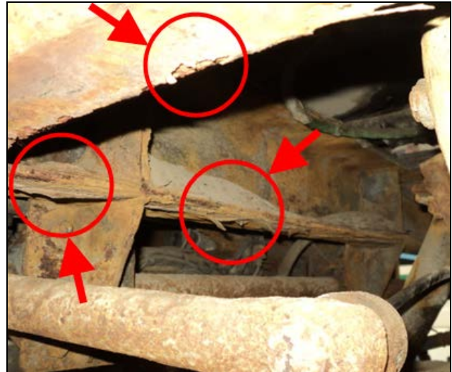
FIGURE 3: METAL FLAKING AND ACCUMULATED SAND
