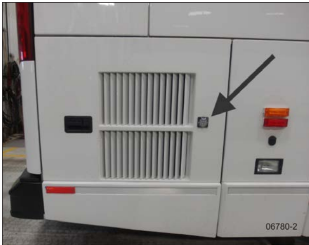
FIGURE 28: BATTERY CHARGER 120-VOLT CONNECTOR
