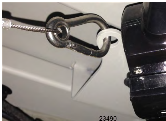
FIGURE 23: PROTECTIVE WIRE INSTALLATION
