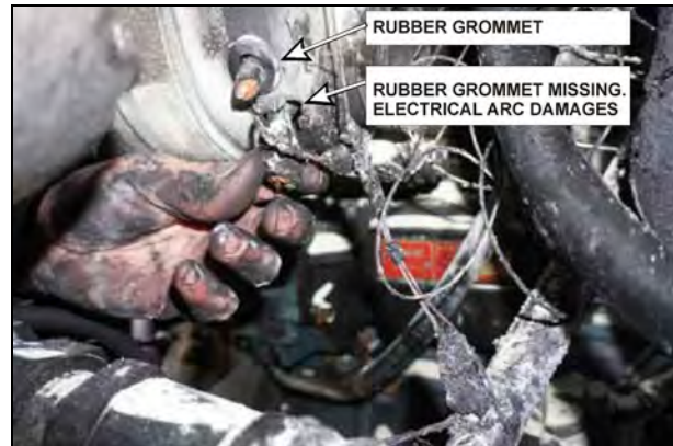
Figure 25: Fire in engine compartment caused by rubbing of power cable against metal edge of Bosch T1 alternator rear cover. Lower rubber grommet was missing when fire occurred. Evidence of electrical arc can be seen.
