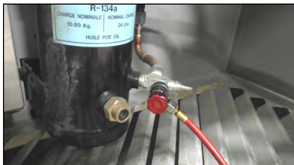
FIGURE 59: RECOVERY UNIT CONNECTED TO RECEIVER SERVICE PORT
