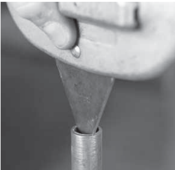
FIGURE 13: DEBURR THE TUBE END - INNER
