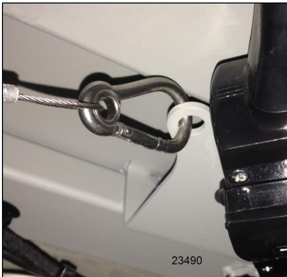
FIGURE 56: PROTECTIVE WIRE INSTALLATION
