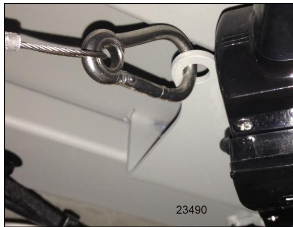
FIGURE 58: PROTECTIVE WIRE INSTALLATION
