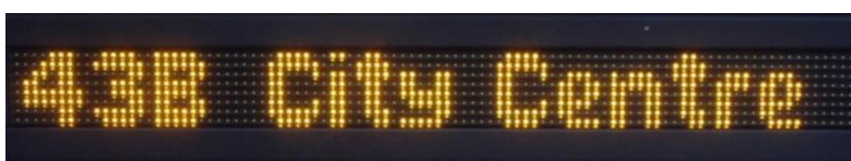
Bypassing a display on a standard communications multi-drop installation
