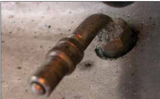
EFFECT: Leaking Valve, Grommet, or Wheel CAUSE: Improper Installation – Torque, Lubrication, Corrosion
