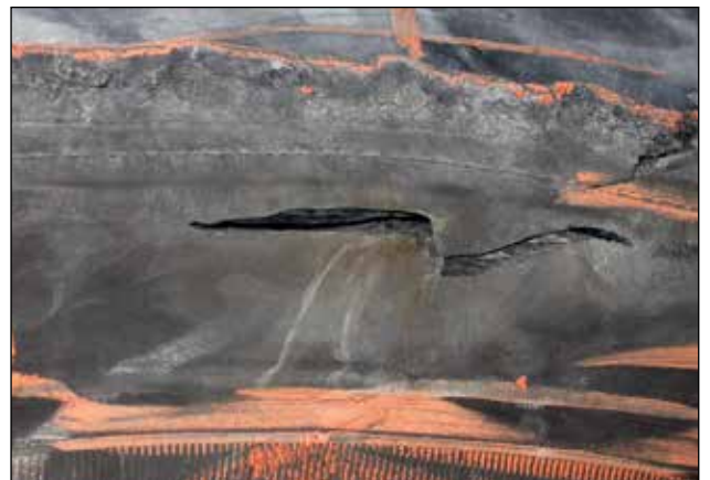
Sidewall Damage from Impact
