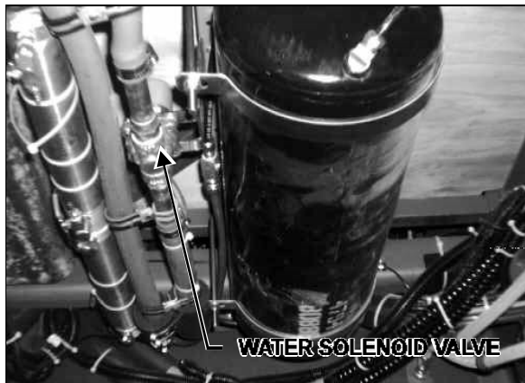
22049 FIGURE 30: CEILING OF THE SPARE WHEEL COMPARTMENT
