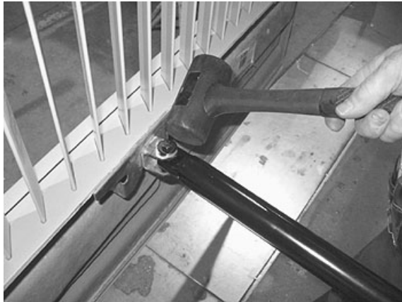
FIGURE 65: DOOR LATERAL ADJUSTMENT
