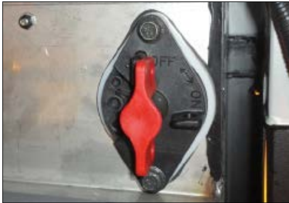
BATTERY MASTER SWITCH
